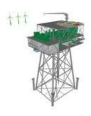
The Borkum 2 wind farm will be developed by BARD Engineering GmbH. It will consist of 80 wind generators of 5 MW located about 130 km from the coast in the North Sea. The generators will feed power into a 36 kV AC cable system which will transformed to 154 kV for the HVDC Light® offshore station. The receiving station will be located at Diele 75 km from the coast where the power will be injected into the German 380 kV grid.
