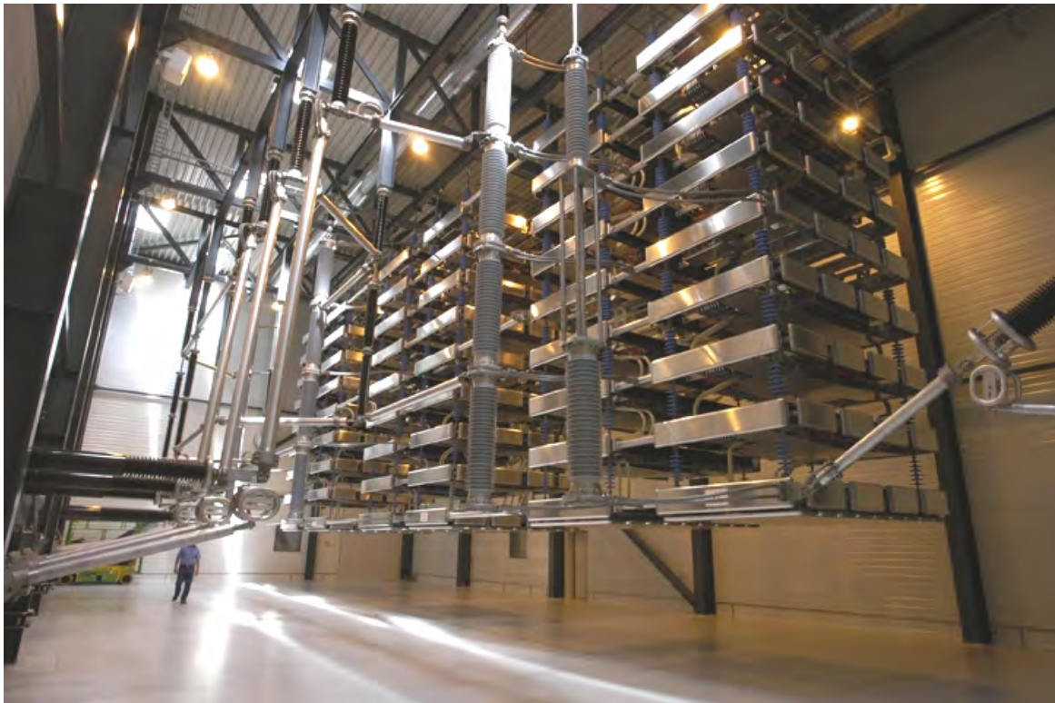
Figure 9.1.2: 12-pulse thyristor based converter inside its valve hall
