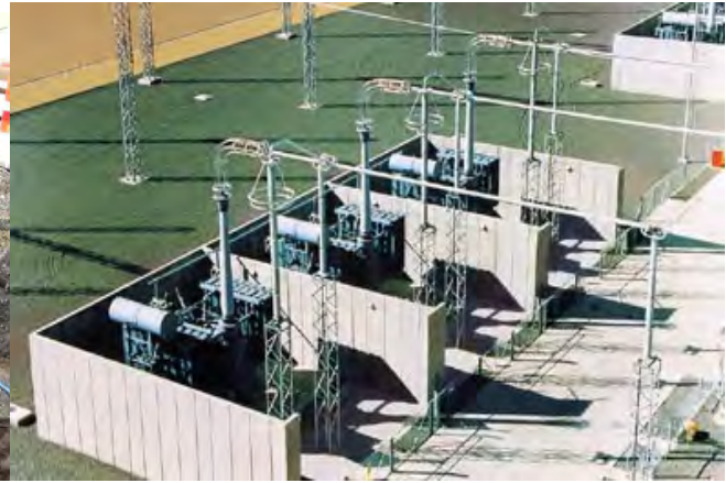
Fig. 7.8(b) Three Single Phase Shunt Reactors
