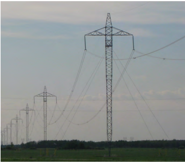
Figure 9.1.10 : Example of use of guyed masts as HVDC transmission structures. Nelson River HVDC Transmission System.
